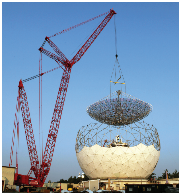
FIGURE 32. The new backstructure is carefully lowered into position on top of the waiting transition structure.
