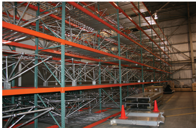
FIGURE 40. Completed subframe trusses await panel installation. All 104 subframe assemblies were stored on racks in an airplane hangar until they were transported to the site.
