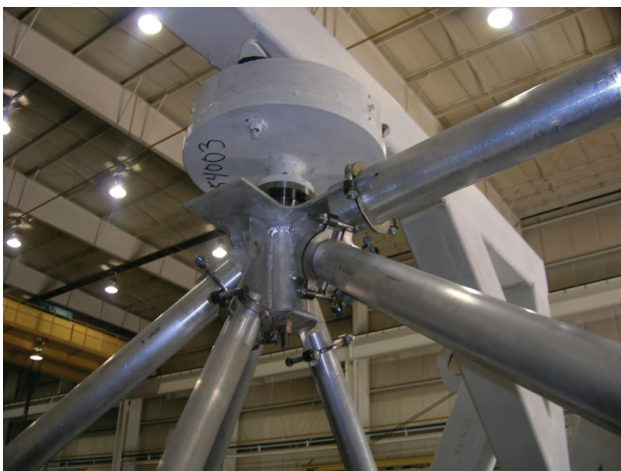
FIGURE A4. Fixturing of backstructure rib tubing to nodes prior to welding operations.
