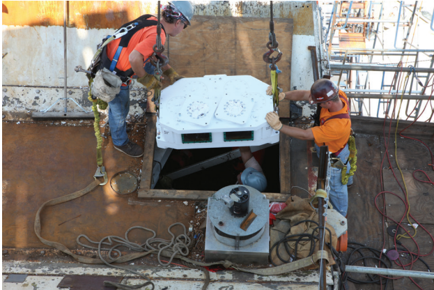
FIGURE 17. The first of the 1-ton gearboxes is lowered into the yoke. The gearbox was then transferred to a series of overhead chainfalls and a rail system in order to position it in place.
