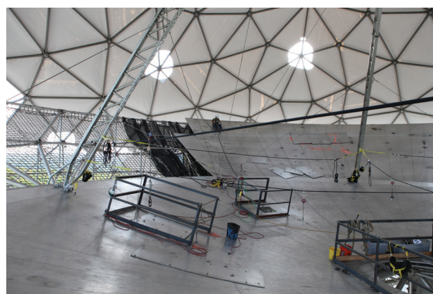
FIGURE 7. (a) Workers remove the first sections of the old antenna surface. (b) Meanwhile, radome membranes are dismantled around the separation line at which the radome will be “uncapped.”
