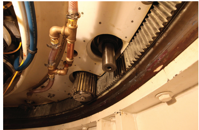
FIGURE 18. One of four pairs of pinions that drive against the stationary 12-foot-diameter bull gear. The shaft on the right is awaiting installation of the pinion gear.
