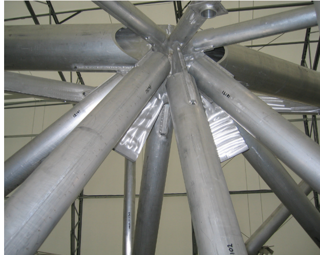
FIGURE 27. This node point has 13 connecting elements.
