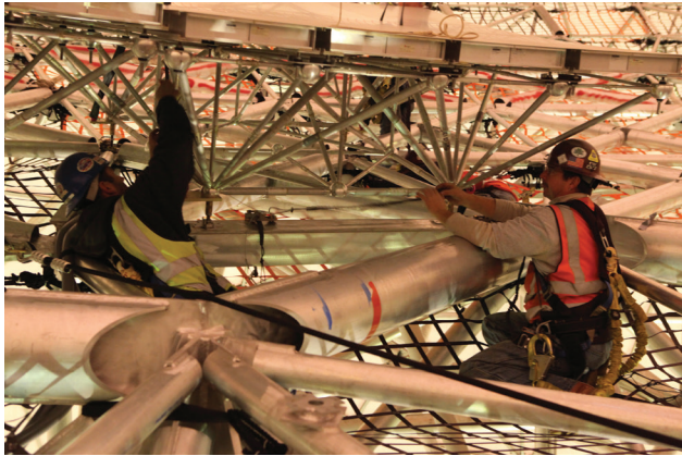
FIGURE 44. Workers in the nets must be careful around the fragile aluminum tubes above and below them.
