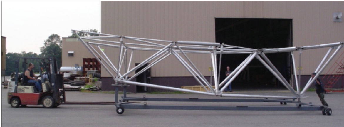
FIGURE A5. Completed radial rib assembly.
