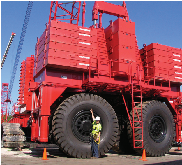
FIGURE 12. The author stands behind the auxiliary counterweight cart while a smaller crane assists with assembling the crane.
