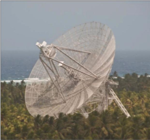
**FIGURE 1.** ALTAIR provides coverage of the deep-space geosynchronous belt, tracking ~1300 deep-space orbiting satellites every week.
