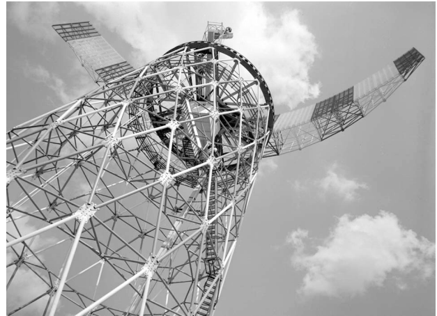
FIGURE 3. Another view of the tower and antenna assembly of the AN/FPS-31 (XD-1) UHF GCI radar. The feed (in the center at the top of the picture) is at the focus of the parabolic-cylinder antenna reflector.
