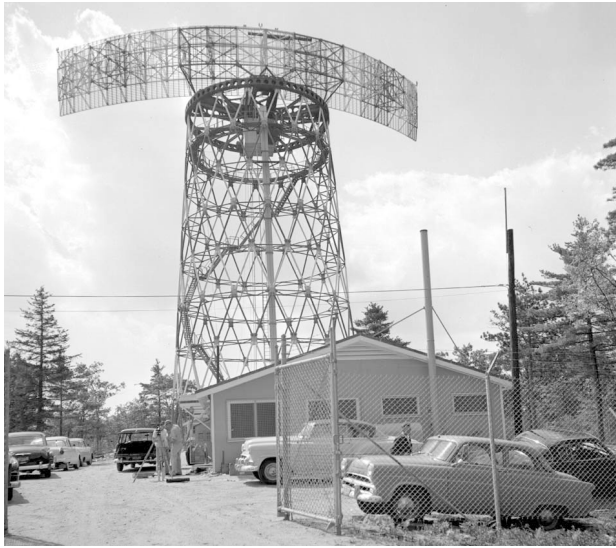
FIGURE 2. The AN/FPS-31 (XD-1) UHF radar at Jug Handle Hill, West Bath, Maine. The vertical waveguide runs from the equipment building to the rotary-joint housing beneath the antenna atop the tower. Note the stairway for scale.
