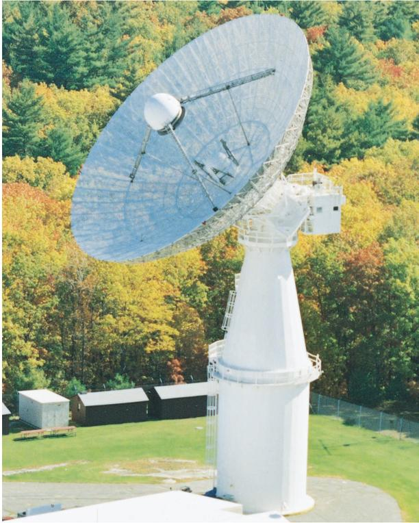
**FIGURE 22.** The Millstone Hill radar in its current configuration in Westford, Massachusetts. Multipulse coherent processing techniques were developed at the Millstone site to enhance the radar’s effectiveness as a deep-space tracking sensor.
