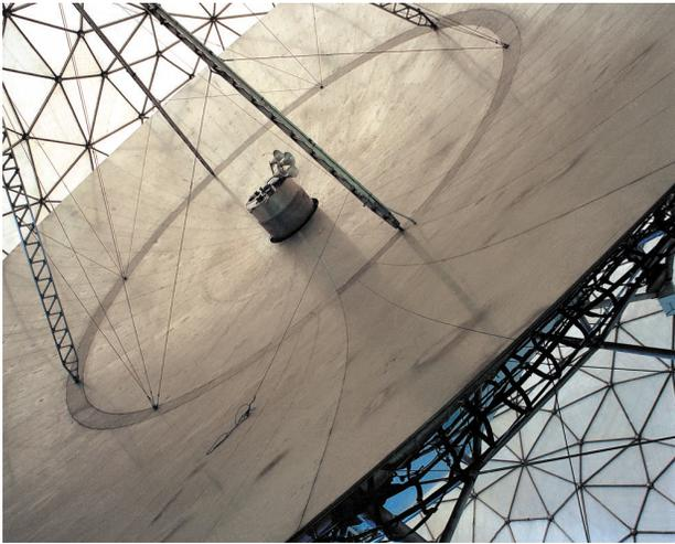
**FIGURE 9.** The Haystack antenna panels and multiple radiometer feedhorns, circa 1994. The feedhorns are mounted on a cylindrical support at the center of the paraboloidal reflector.
