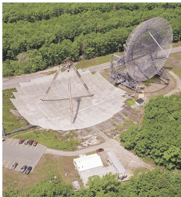
**FIGURE 7.** UHF antennas for ionospheric measurements at Millstone Hill. The fixed 220-ft zenith-pointing antenna (left) was installed in 1963 and the steerable 150-ft-diameter antenna (right) was installed in 1977.
