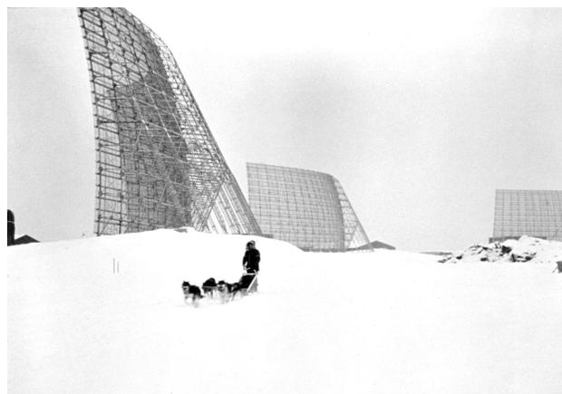
**FIGURE 2.** Three Ballistic Missile Early Warning System (BMEWS) AN/FPS-50 surveillance radars at Clear, Alaska. The parabolic-torus antenna reflector of an AN/FPS-50 radar was approximately the size of a football field.
