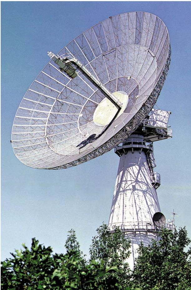
**FIGURE 3.** The UHF Millstone Hill radar with its reflector and scanning feed, circa 1958. Located in Westford, Massachusetts, the Millstone system included an 84-ft paraboloidal reflector and conical feed mounted on an elevation-angle-over-azimuth pedestal and a klystron transmitter operating at UHF with 1-MW peak and 60-kW average power.
