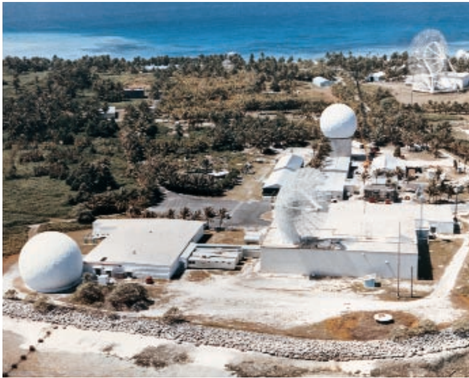
FIGURE 3. The Kiernan Reentry Measurement System (KREMS) facility located on Kwajalein Atoll in the central Pacific Ocean. The ALCOR C-band radar is located under the white radome in the lower left of the photograph. The millimeter-wave radar is located under the smaller white radome near the center.
