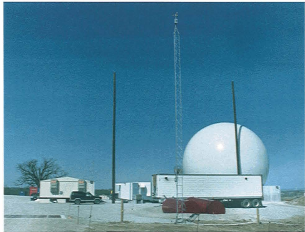
FIGURE 3. TDWR testbed located southwest of Kansas City International Airport.
