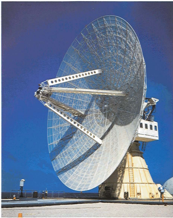
FIGURE 3. The TRADEX parabolic antenna is 25.6 m in diameter. Its two-way 6-dB beam width is 10.6 mrad, or 0.61^\circ , which is slightly larger than the angular width of the moon.
