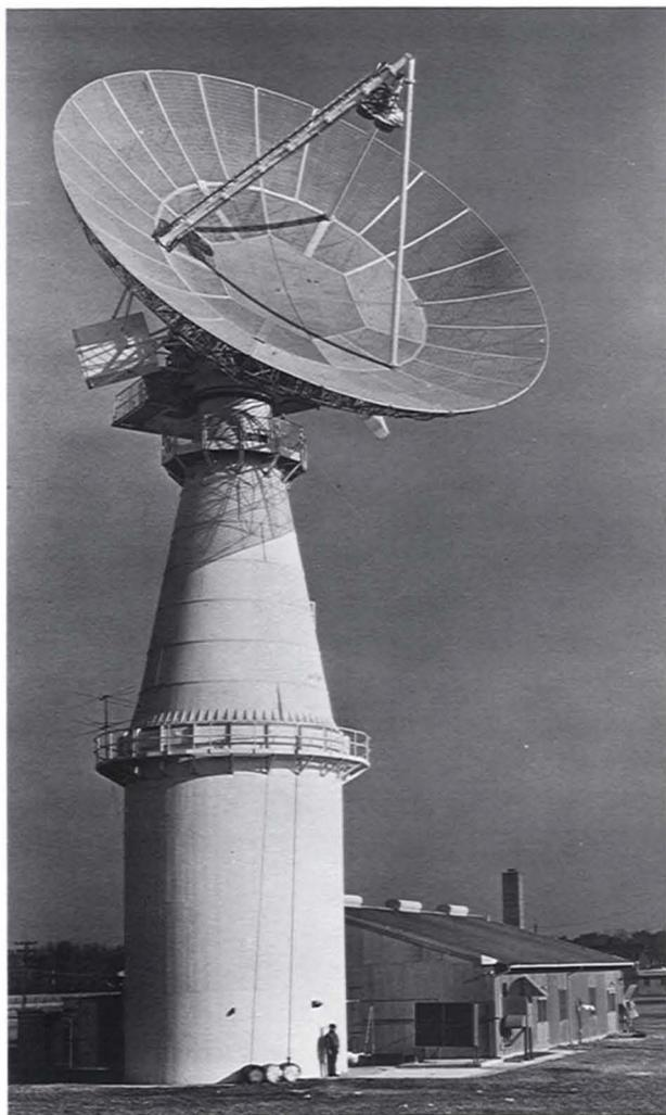
**FIGURE 2.** The 60-ft antenna and mount of the SPANDAR S-band tracking radar designed by Lincoln Laboratory for NASA.
