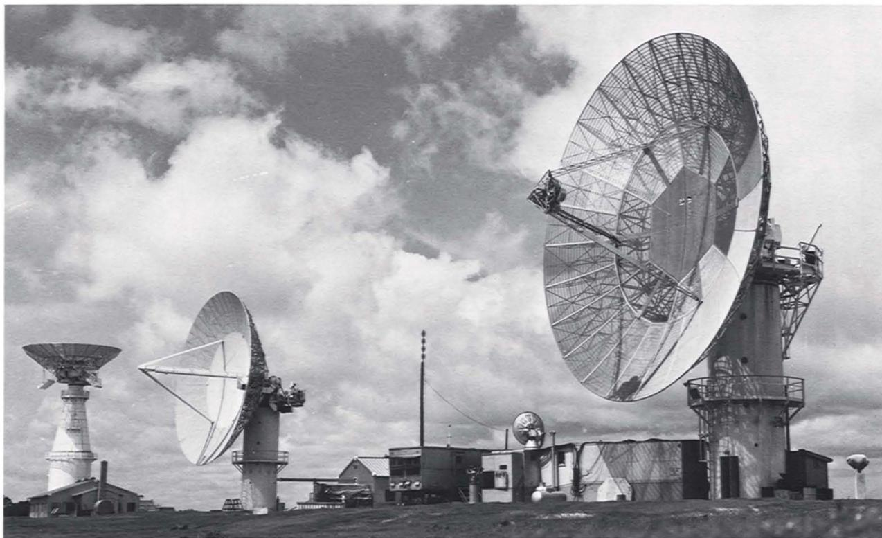
**FIGURE 1.** Radar antennas at the Lincoln Laboratory field site at Arbutle Neck, Va., located near the NASA Wallops Island launch facility. Site instrumentation consists of (from right to left) the S-band tracking radar, the multiplexed UHF and X-band cross-section measurements radar, and the SPANDAR long-range trajectory and range-safety radar designed by Lincoln Laboratory for NASA.
