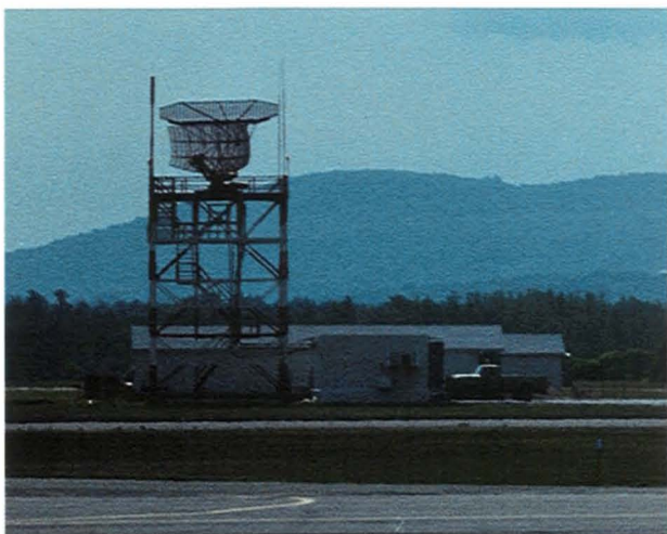
Fig. 7—The ASR-7 radar at Burlington, Vt., used for testing the Moving Target Detector (MTD). The surrounding hills provided a high-clutter environment to test and demonstrate the clutter reduction capability of the MTD.
