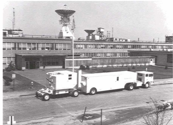
Fig. 6 — Lincoln Experimental Terminal (LET)-1 — a complete, self-sufficient, transportable terminal for SHF space communications — ready to roll.
