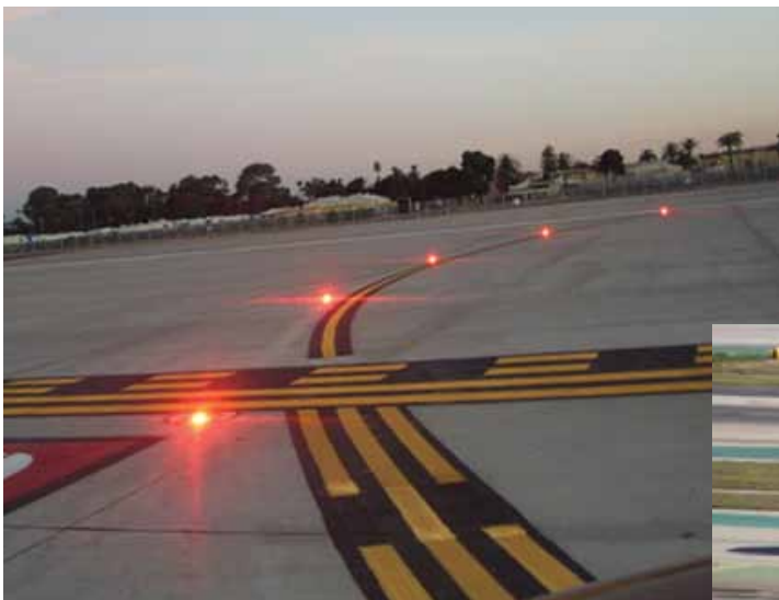
Lincoln Laboratory has supported the FAA in developing and deploying the Runway Status Lights system at the Los Angeles International Airport. The system includes Takeoff Hold Lights and Runway Entrance Lights at key locations to reduce the potential for runway incursions.
