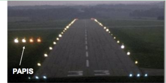
Precision Approach Path Indicator (PAPI)
