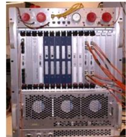
COTS Modular Processor Beamformer
