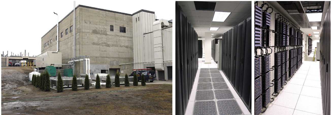
FIGURE 22. Building F and the shared computing facility, built to provide space for Lincoln Laboratory's computing resources. The building supplies the necessary power and cooling to house a large number of computers and provides infrastructure for collateral compute resources. The LLGrid system was moved into Building F in the spring of 2006.
